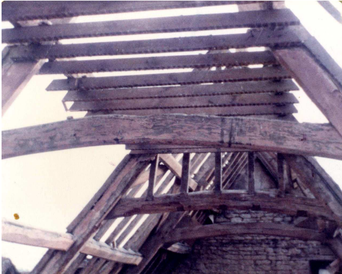
Original roof structure in c.1980: 3 trusses, the centre one with stud partition
