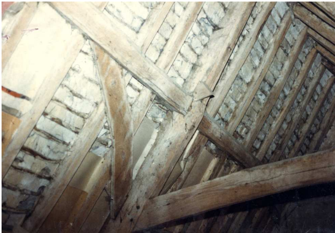
Detail of original roof structure in c.1980, with tenoned purlins and wind-brace
