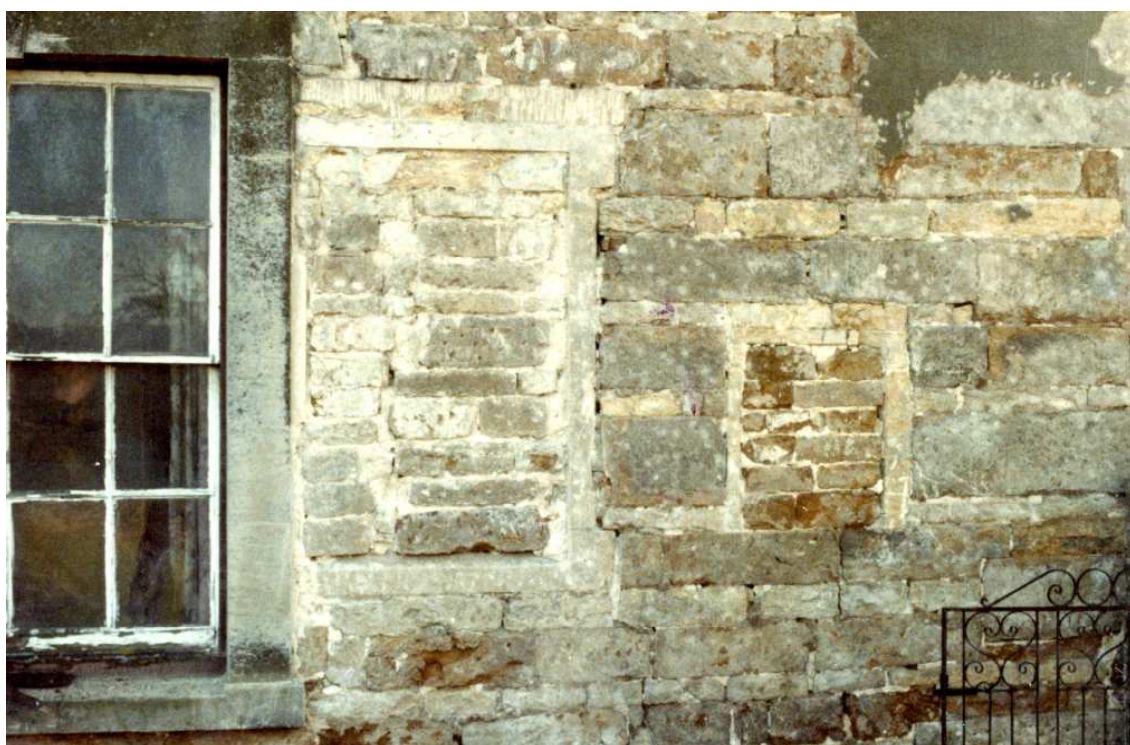
Blocked original windows to south end of west front in c.1980
